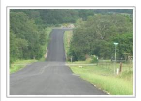
Lution Road improvements project included replacement and widening of the existing pavement and improvement of two 90 degree curves to improve safety.
