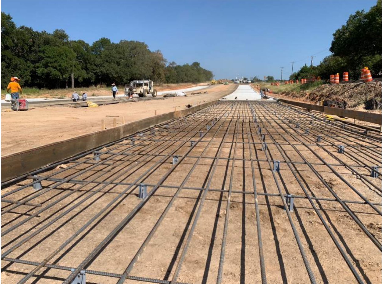
Eastloop Phase 1 – steel placed for tie in at IH-20
