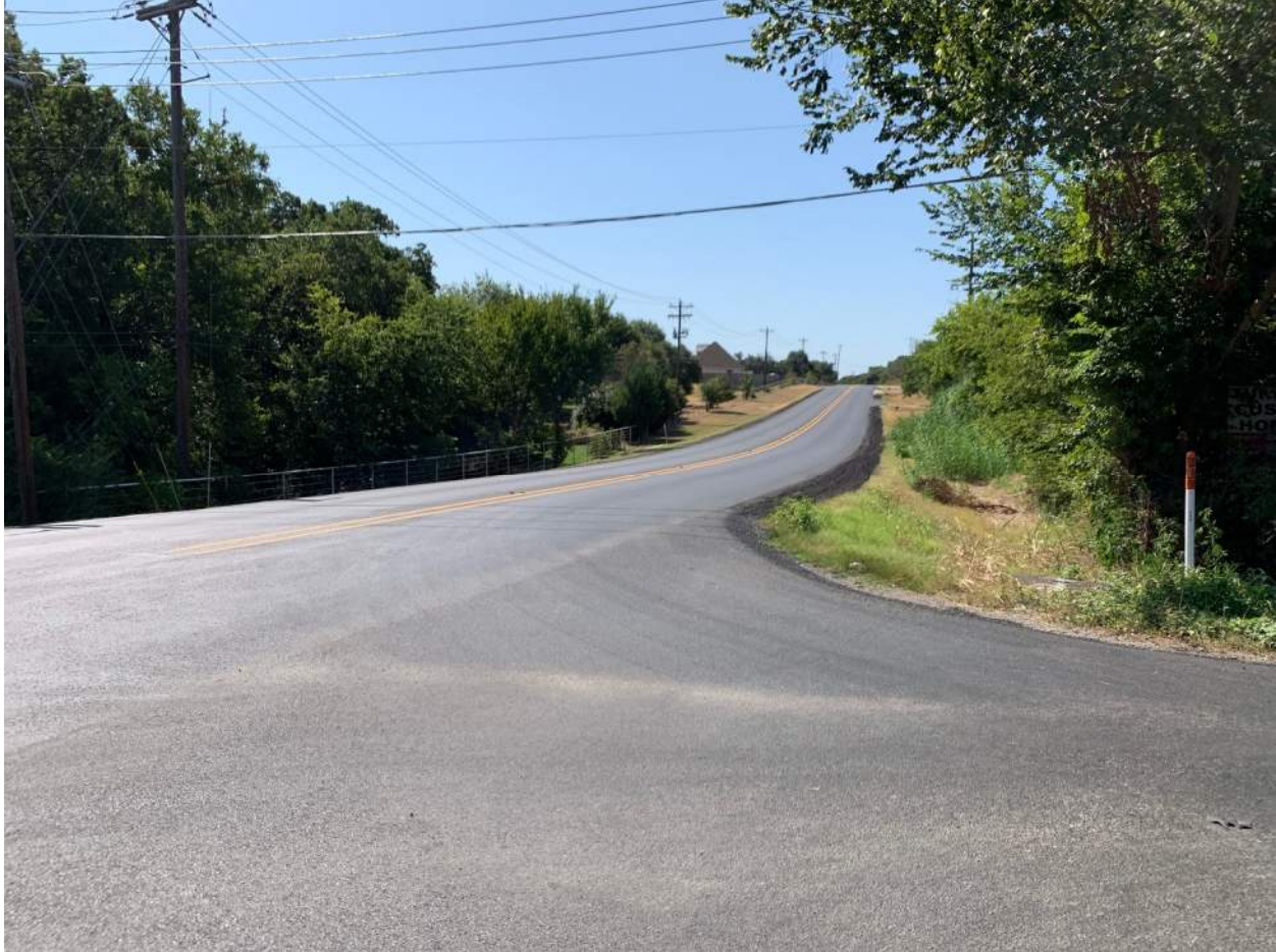
FM 5 – Overlay completed
