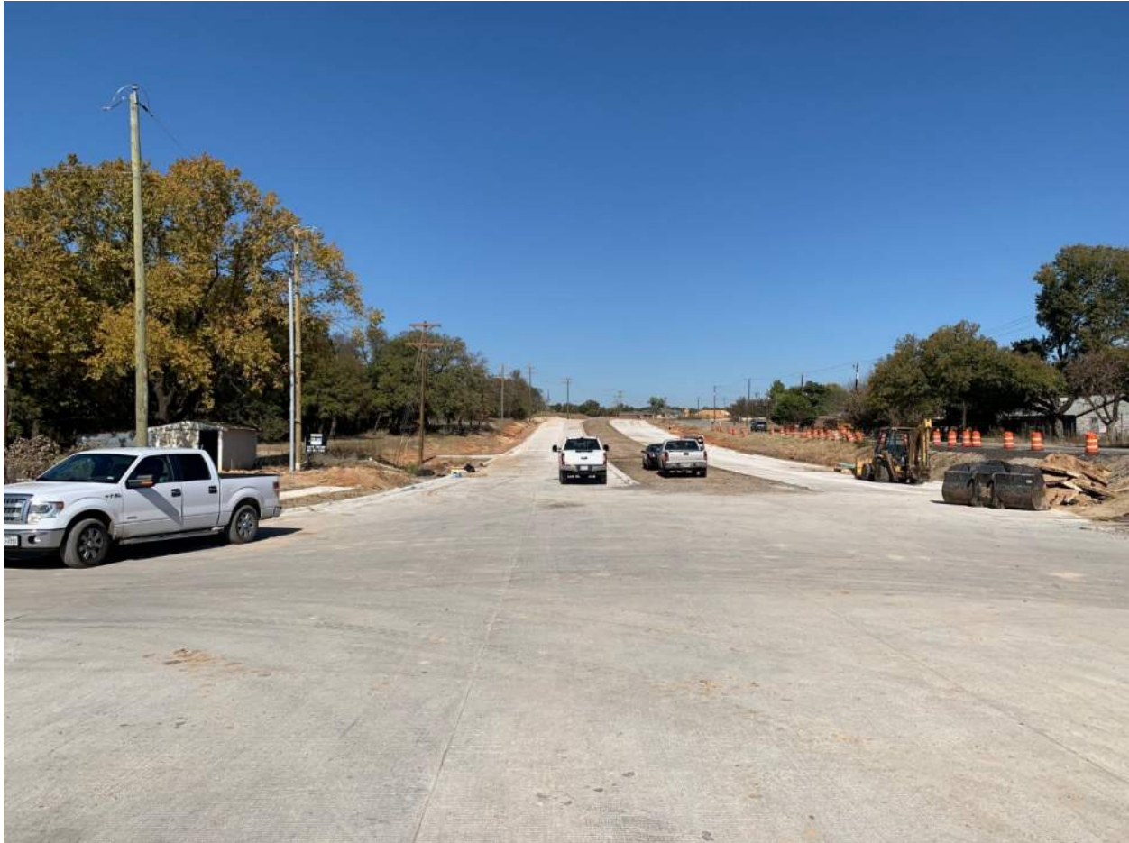
Eastloop Phase 1 – tie in at IH-20 complete
