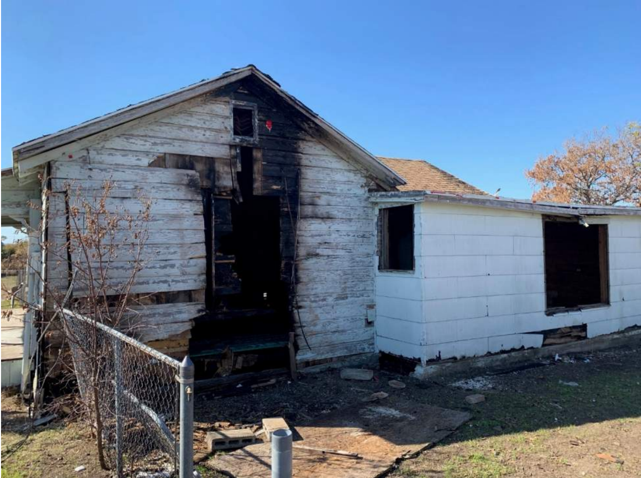
House demoed on Parcel 100
